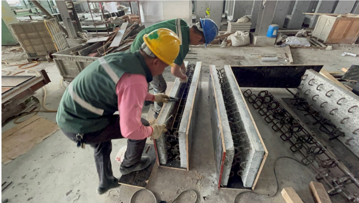
Installation of the middle rebars
